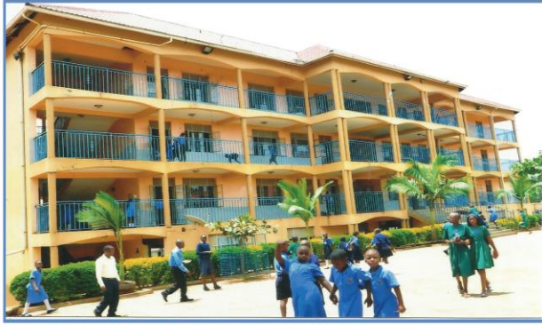
The Main Classroom Block
