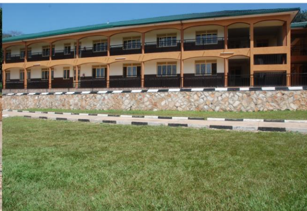
Modern facilities constructed in 2016
