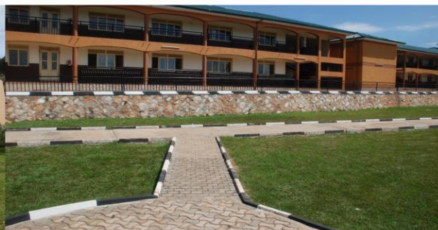
Modern facilities constructed in 2016
