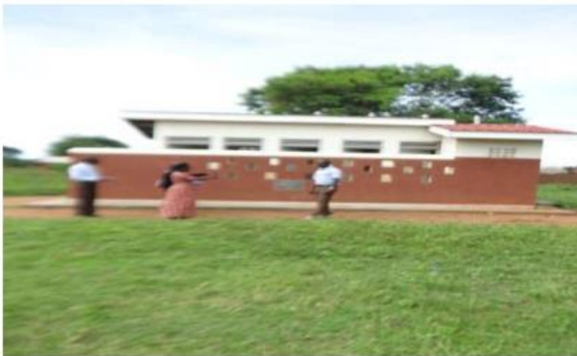
A brief inspection of one of the five Ventilated Improved Pit Latrines.
